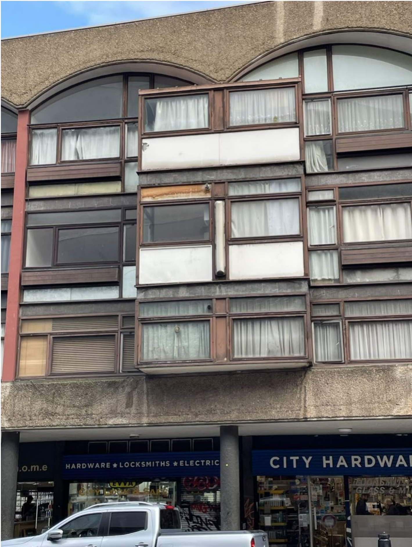
Image 1 – Crescent House, Western Elevation (facing Goswell Road)
