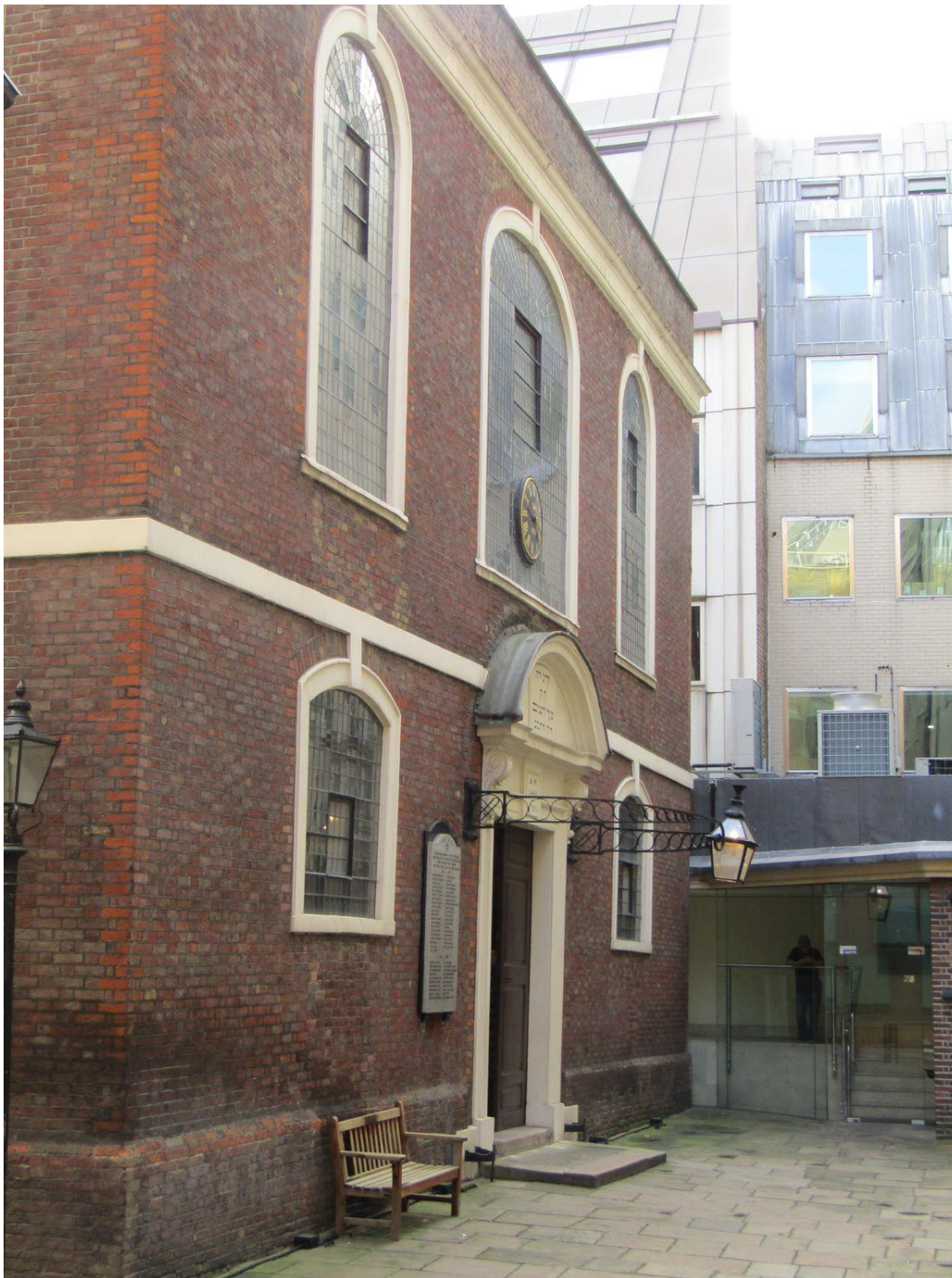
Figure 7: Bevis Marks Synagogue, western elevation
