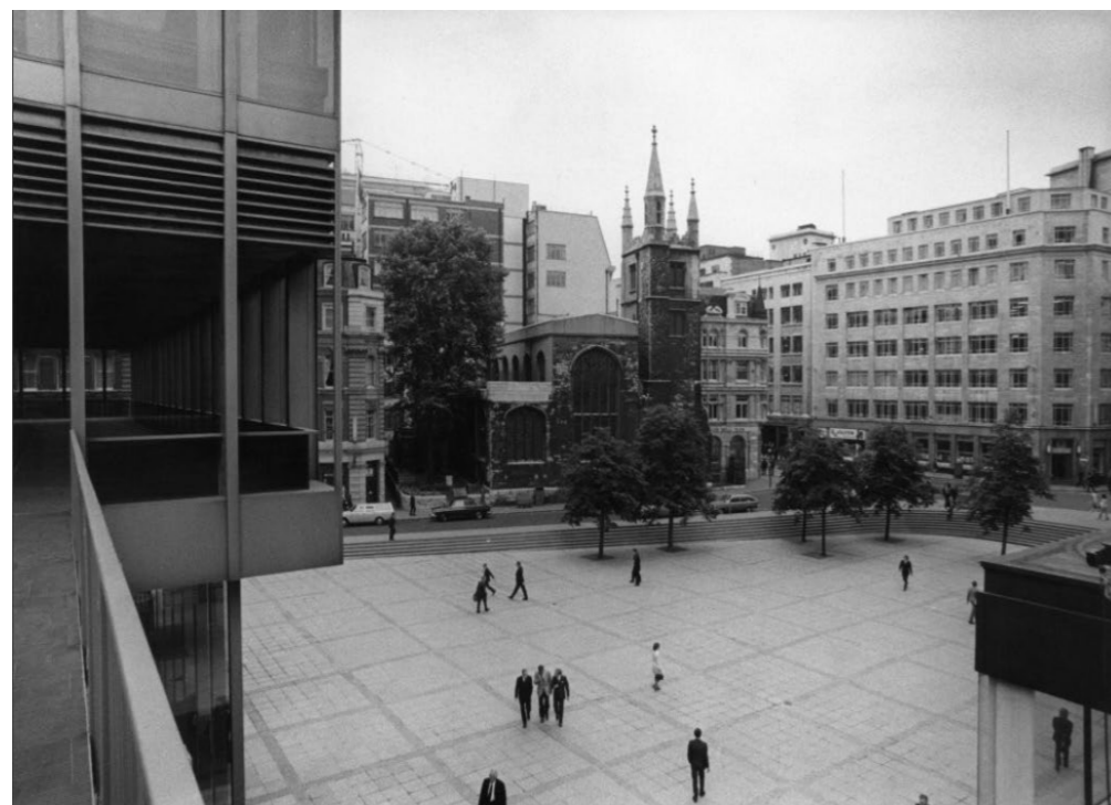
Figure 7: 1973 Commercial Union Tower (Aviva Tower), 1 Undershaft, City of London: the pedestrian walkway leading into the first-floor of the building (podium level), linking to the P&O building. Source: RIBA Ref No RIBA121146.
