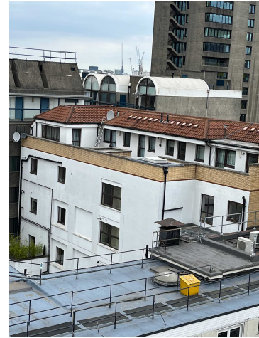
Bridgewater House close up
