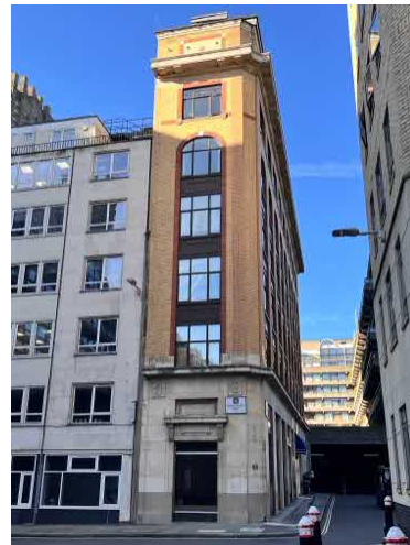
Bridgewater House, eastern elevation
