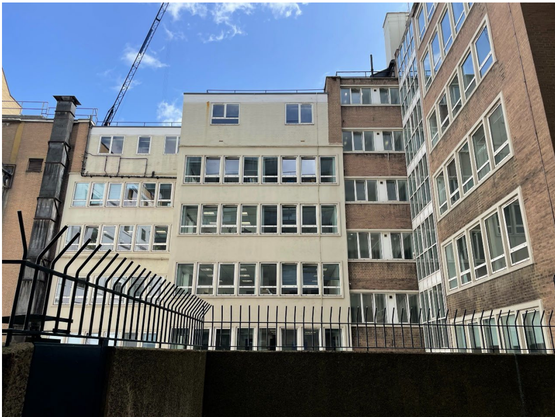
Image 4: View of westerly facing internal courtyard elevation
