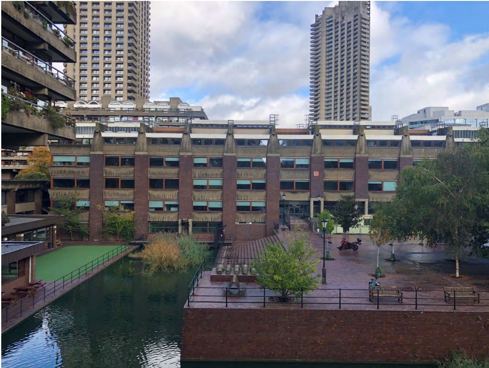
View from Wallside (Figure G)
