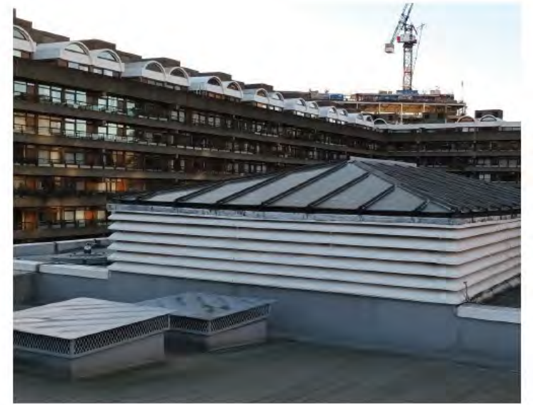
Fig 2: View b of East Elevation, looking South West towards Thomas Moore House
