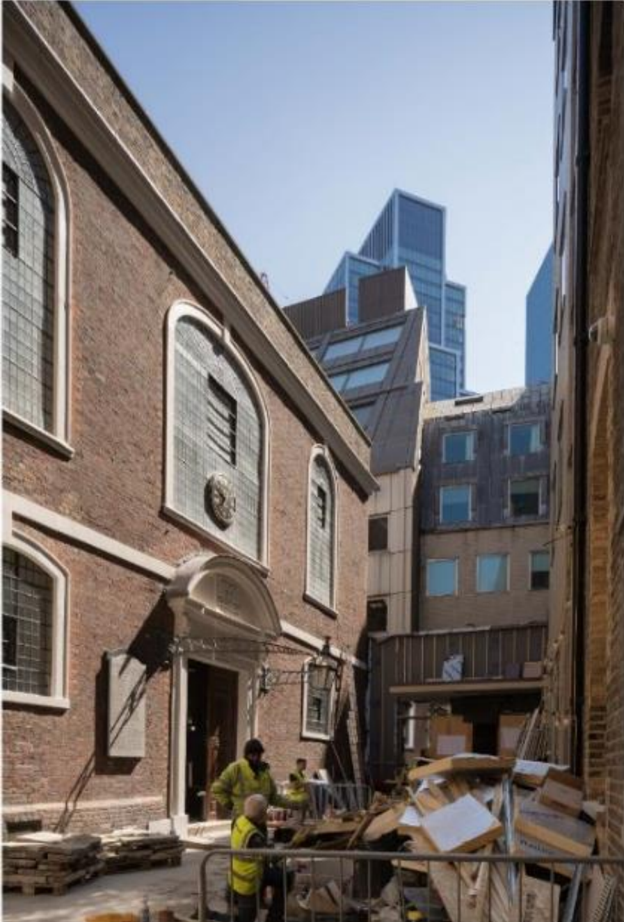
Existing View – View 45a
