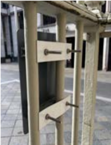
Fig. 108 Crude fixings to CoL sign, 2024
