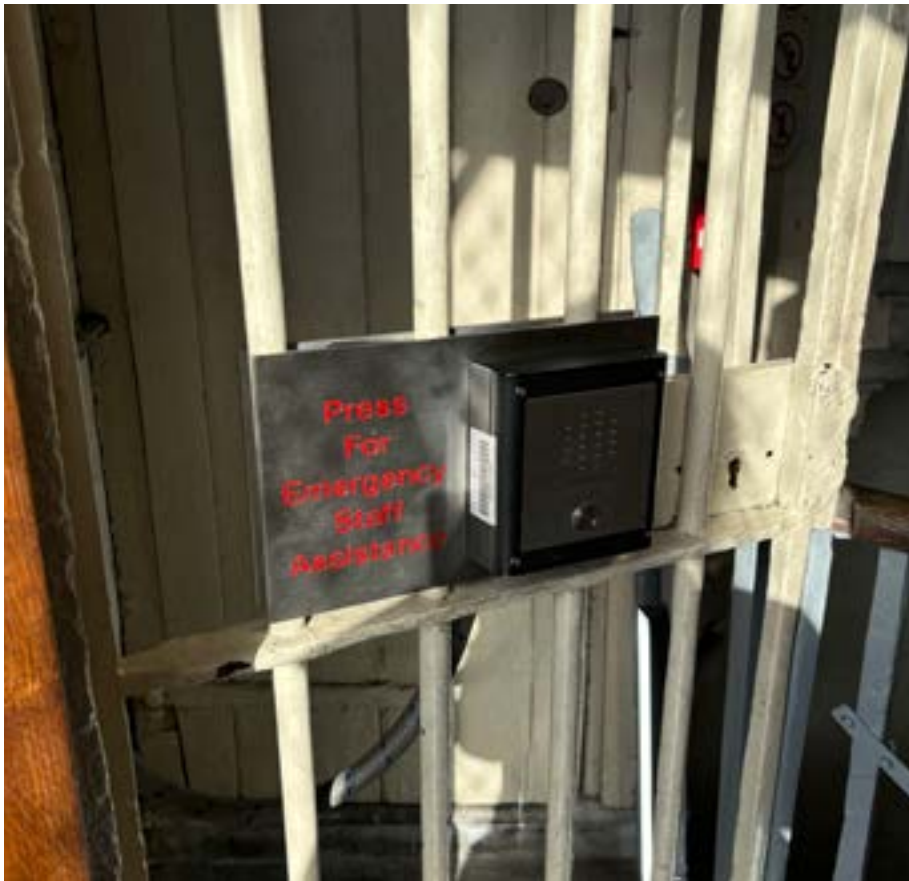
Fig. 92 Viewing platform intercom connecting to ground floor reception, 2024
