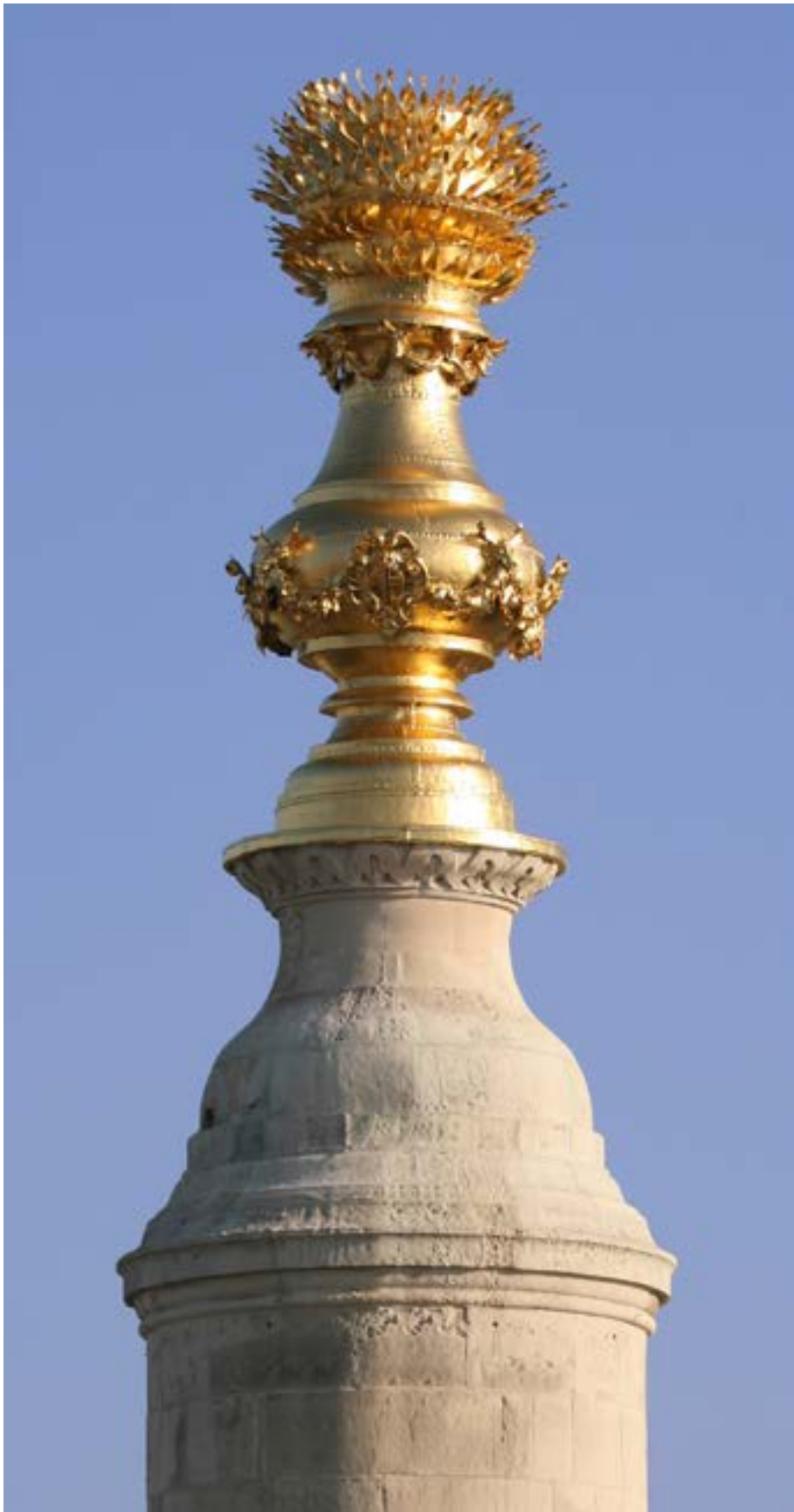
Fig. 47 The gilded copper flaming orb on the stone dome and drum 2009
