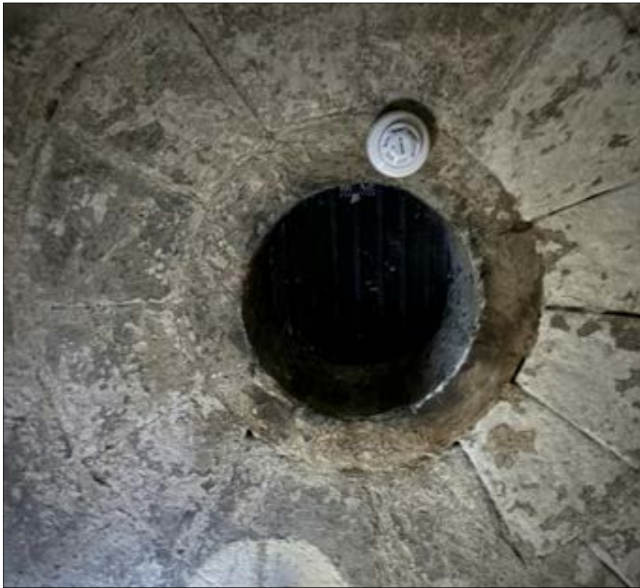
Fig. 67 Central circular basement room, looking up at the (blocked-up) oculus in the stone domed soffit, 2024
