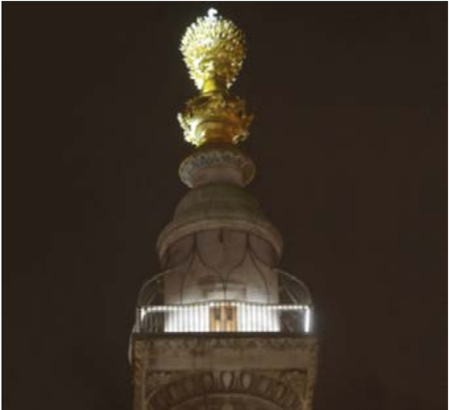
Fig. 117 LED rope to underside of balustrade handrail, 2018
