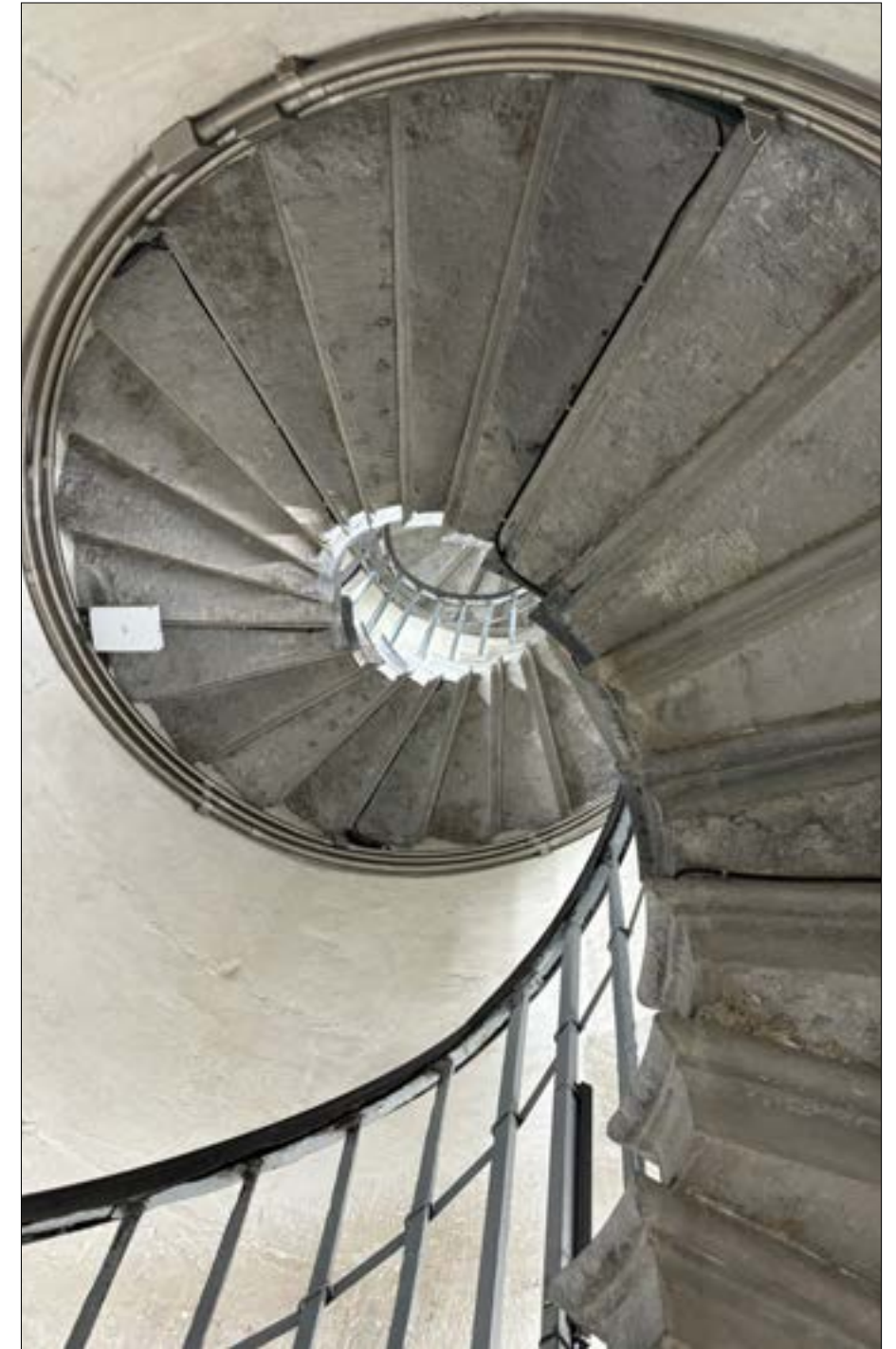
Fig. 60 Looking up at the underside of the stair treads at the original black limestone, 2024
