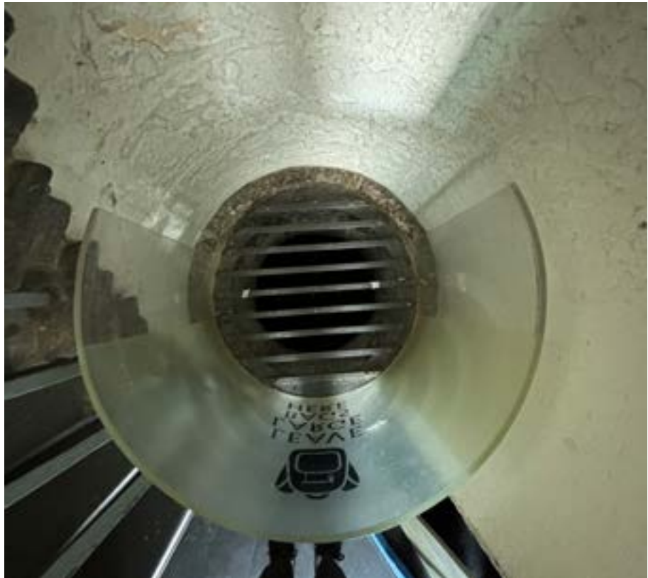
Fig. 84 Circular wrought iron grille at the basement dome oculus/base of helicar stair, 2024
