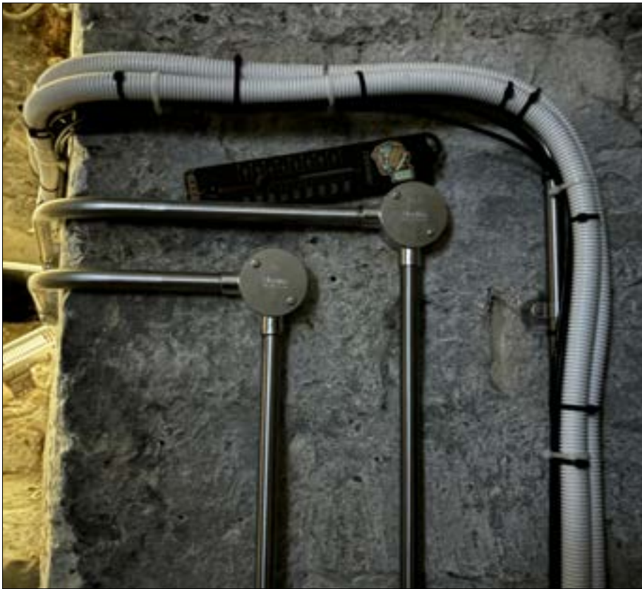
Fig. 68 Neat stainless-steel conduits & junction boxes, and temporary Cat6 cables to basement computer (for redundant Panoramic camera installation), 2024
