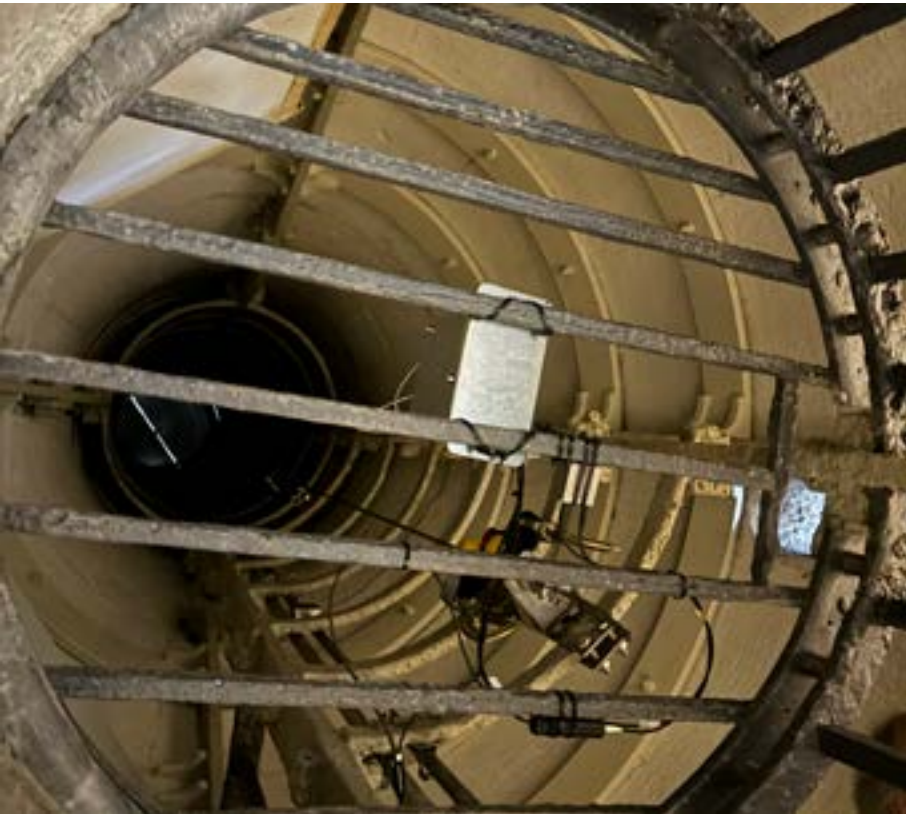
Fig. 82 Circular wrought iron grille at the base of the flaming orb armature, 2024
