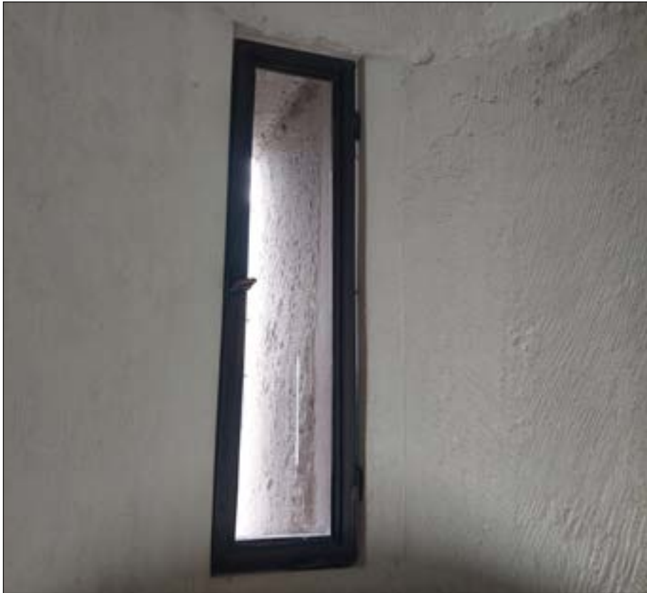
Fig. 51 Bronze casement window flush with stone wall, 2024
