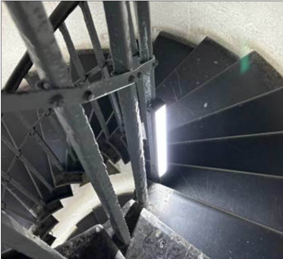
Fig. 70 Replacement stairwell lighting, 2024
