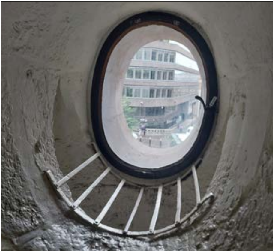
Fig. 54 Iron oval casement window, 2024
