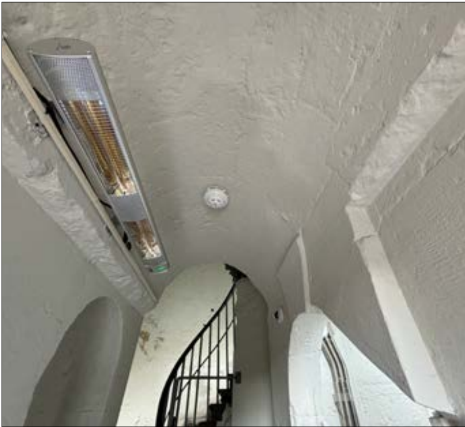
Fig. 72 Entrance foyer showing heater, redundant strip-uplighter, smoke detector, CCTV camera, stainless-steel conduits, 2024.
