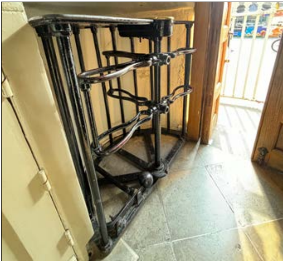
Fig. 63 c.1891 turnstile with the projecting ‘arms’ and the central rail temporarily removed (north side), 2024.
