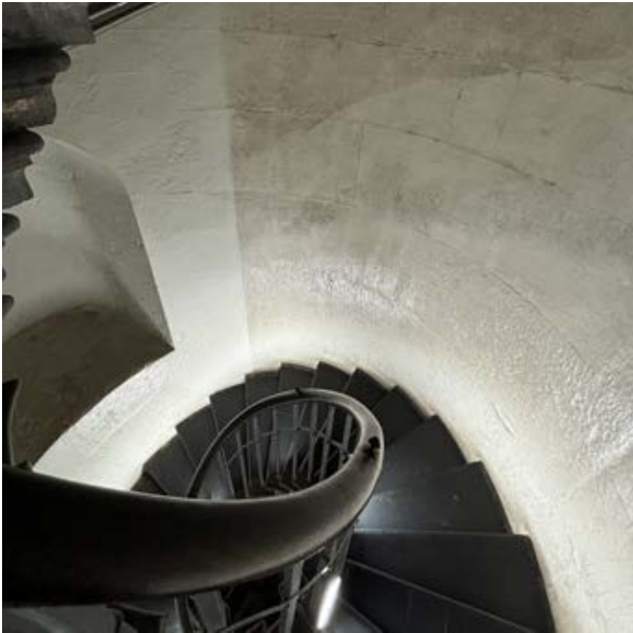
Fig. 85 Staircase balustrade curved oak handrail, 2024
