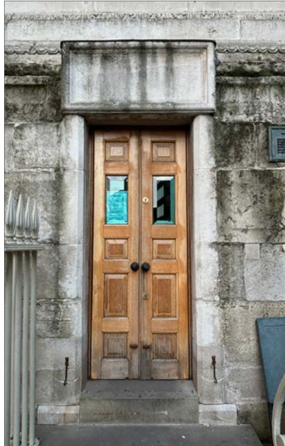
Fig. 55 Pair of glazed oak entrance doors, installed 2009, 2024.
