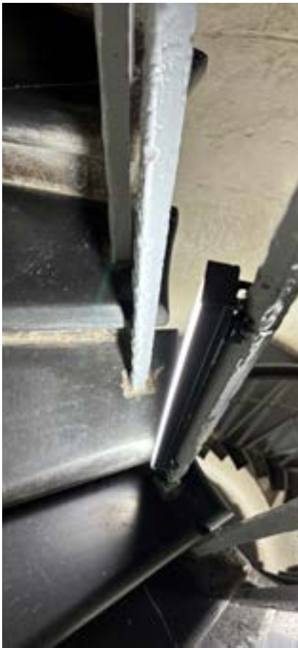
Fig. 97 Replacement light strips
