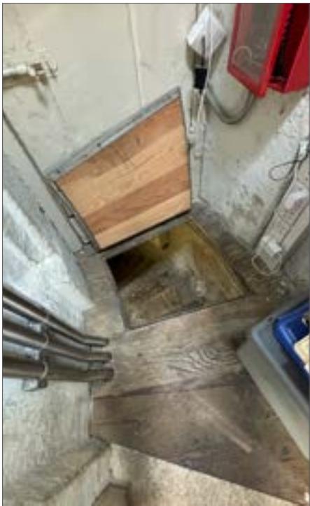
Fig. 55 Floor hatch access to the basement, 2024
