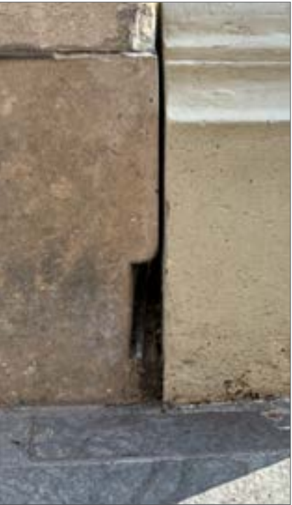
Fig. 119 Drainage gap from south Area to surrounding paving, 2024
