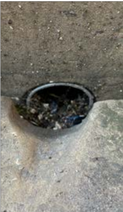
Fig. 116 Close-up blocked pipe, 2024
