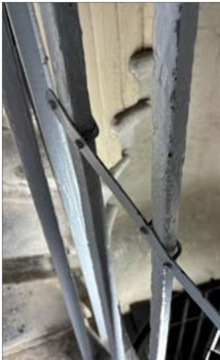
Fig. 39 Steel flat clasped to balusters, 2024
