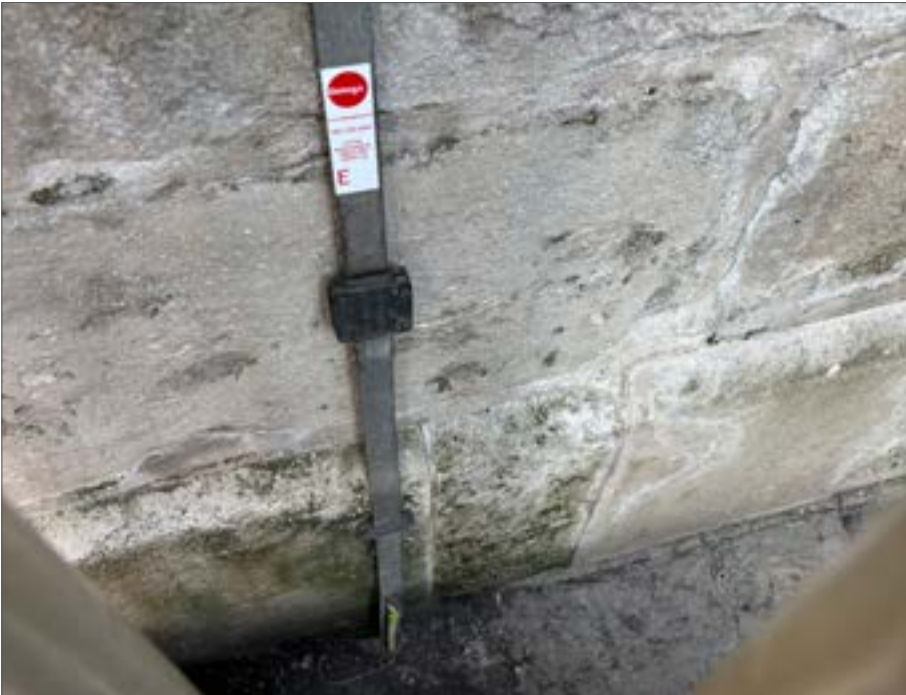
Fig. 109 East elevation down conductor, surface mounted, 2024
