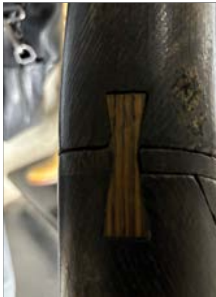
Fig. 46 Recent unstained butterfly joint, 2024
