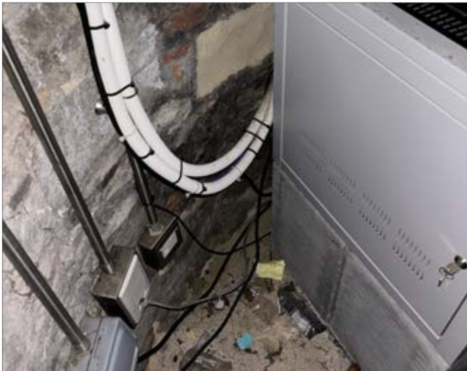
Fig. 82 Debris and redundant wiring in the central circular basement, 2024
