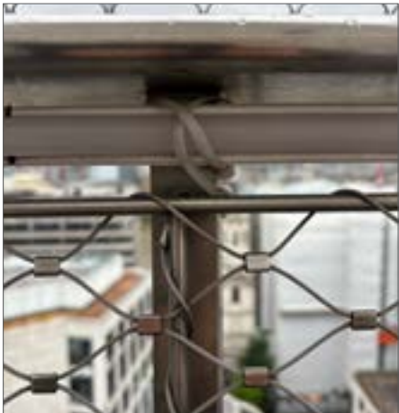
Fig. 90 A rope of LED lights fixed to the underside of the handrail, 2024
