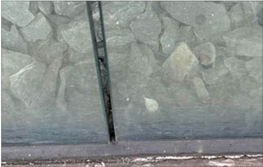
Fig. 120 Open joints between structural glass, 2024
