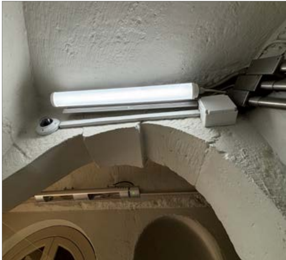
Fig. 104 Replacement light fitting, plastic conduit and junction box, 2024
