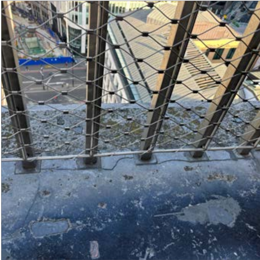
Fig. 12 Crack line along the base of balusters, 2024
