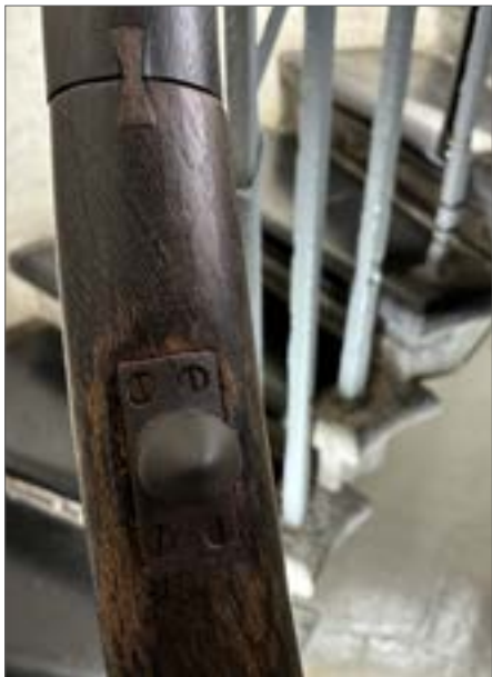
Fig. 44 Brass 'anti-sliding' knob, 2024
