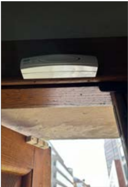
Fig. 27 Door movement detector, 2024
