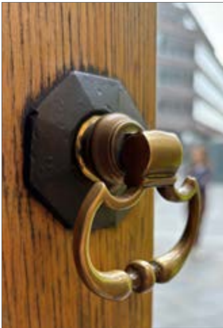
Fig. 26 Mortice interior escape latch, 2024
