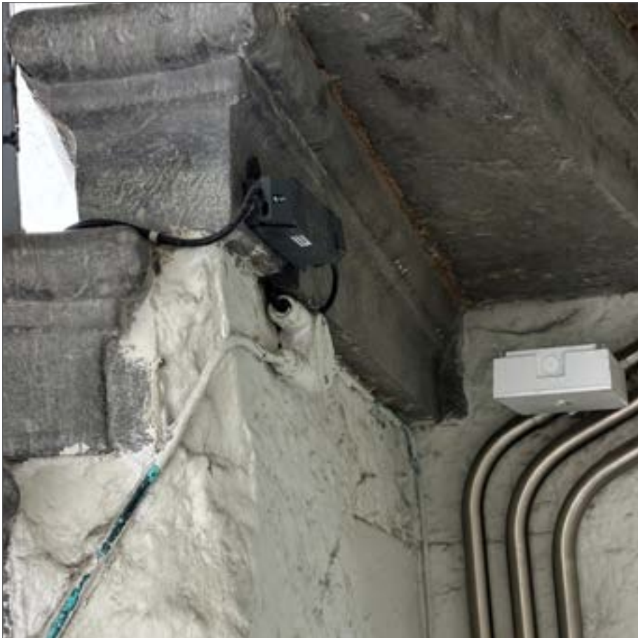
Fig. 101 White emergency light and black transformer, 2024
