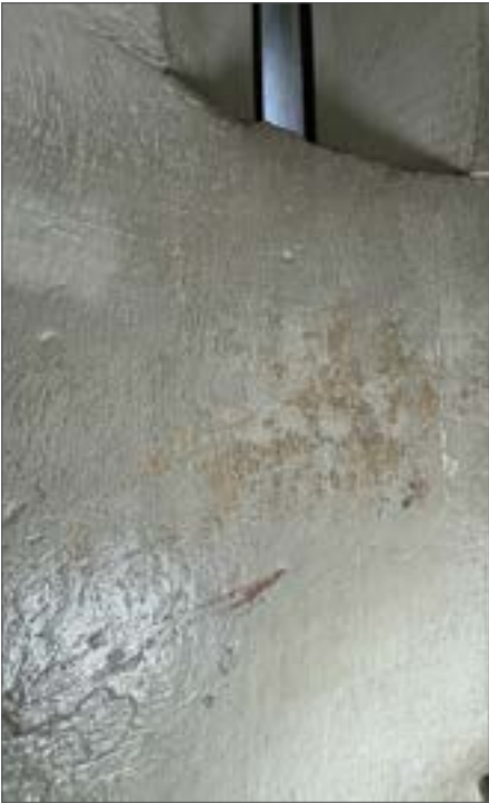
Fig. 32 Eroded paintwork, 2024
