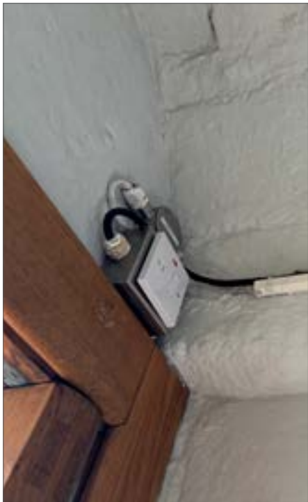
Fig. 86 Power supply and isolator, 2024
