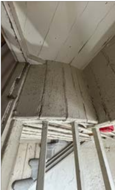
Fig. 51 Balusters lead-caulked into treads, 2024
