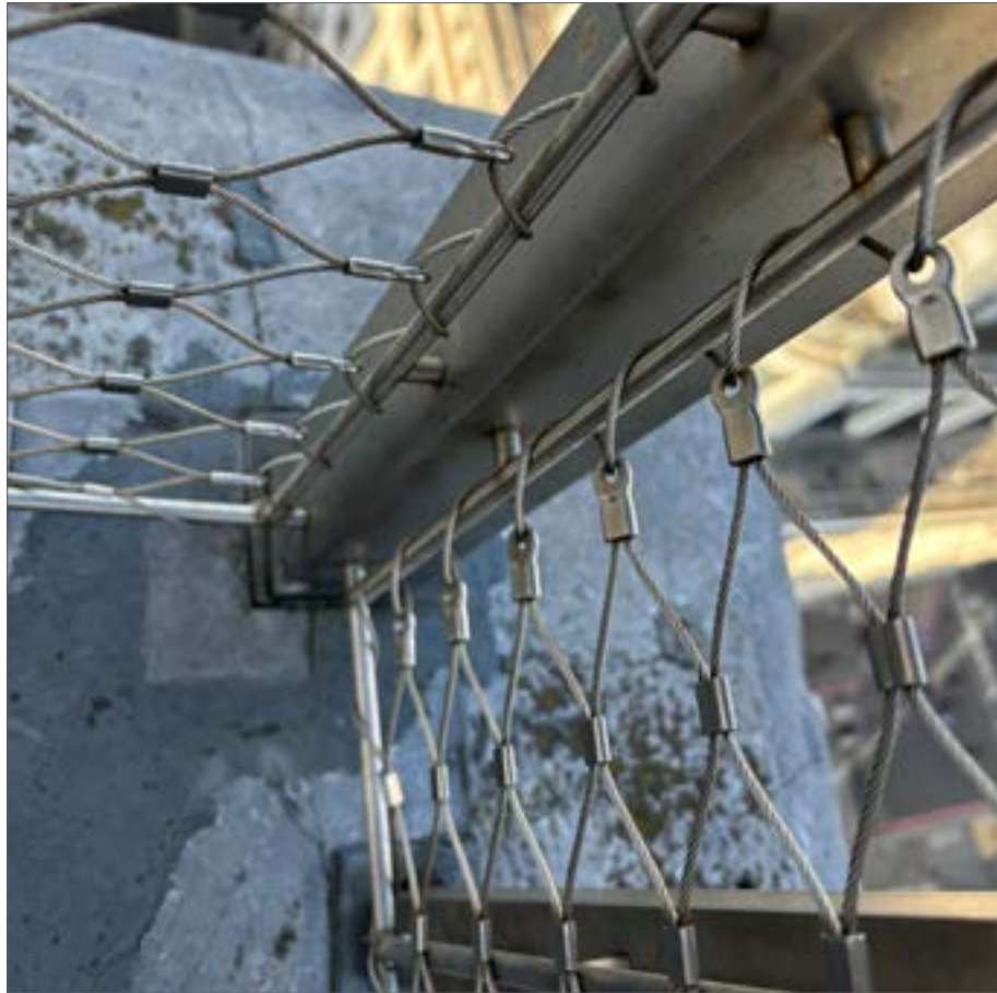
Fig. 13 Detail of a balustrade corner post, 2024
