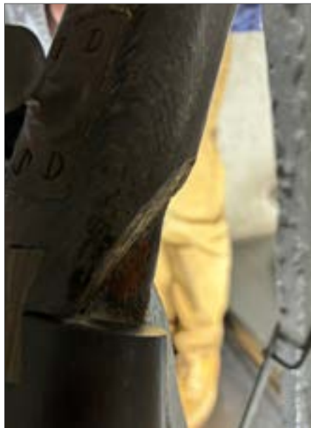
Fig. 45 Damaged section of handrail, 2024
