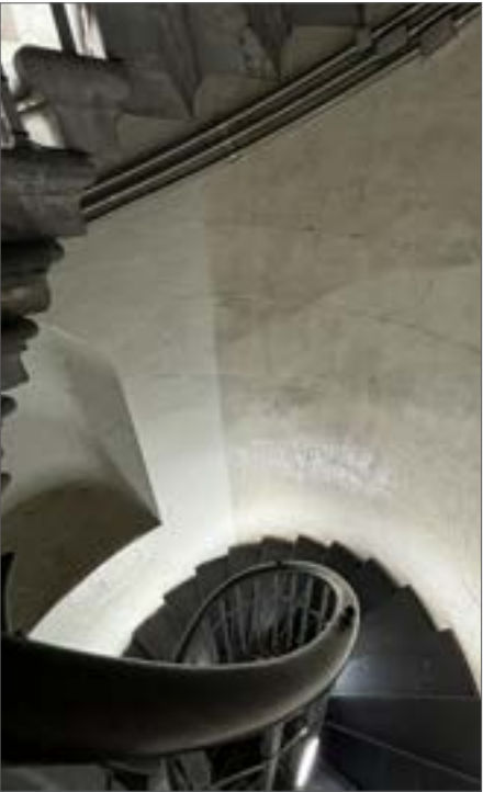
Fig. 30 3 wall finishes: repainted walls at bottom of stairwell; upper stair is cleaned to head-height, then dirty above, 2024
