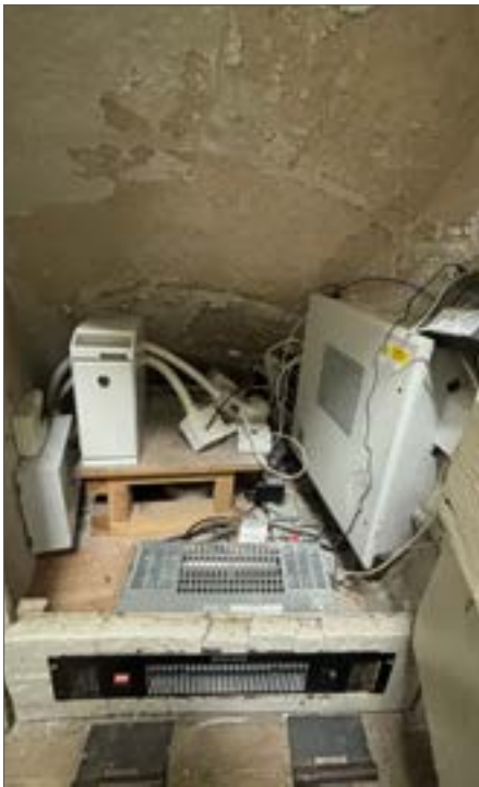
Fig. 87 Kick-space fan heater in skirting of cupboard, 2024
