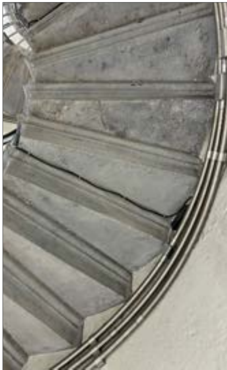
Fig. 37 Underside of one step is in markedly poorer condition, 2024
