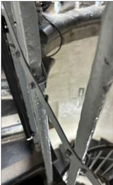
Fig. 40 Steel flat bends around baluster , 2024
