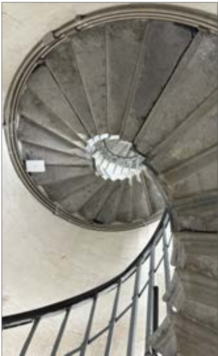
Fig. 36 Underside of stairs with pocket in stonework of central tread, 2024
