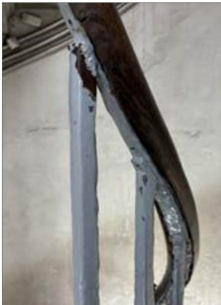
Fig. 43 Fixing of timber to ironwork, 2024
