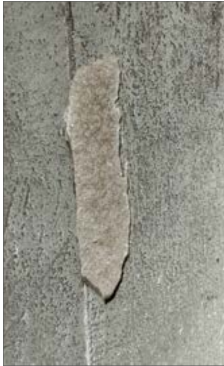
Fig. 33 Local spalling of stonework, 2024
