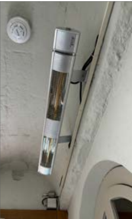
Fig. 84 Radiant electric heater, black cabling is visible, 2024
