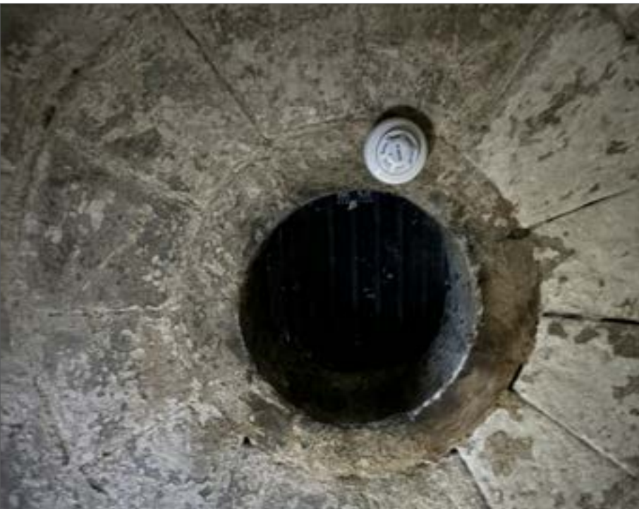
Fig. 81 Blocked-up oculus opening at the apex of the basement vaulted soffit, 2024
