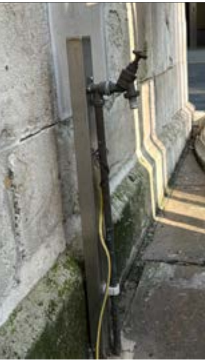
Fig. 114 Tap, with earthing cable, 2024
