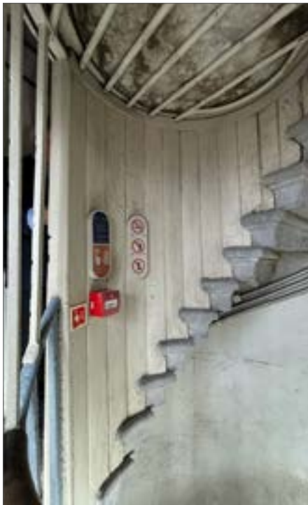
Fig. 50 Steel flat bends around baluster, 2024
