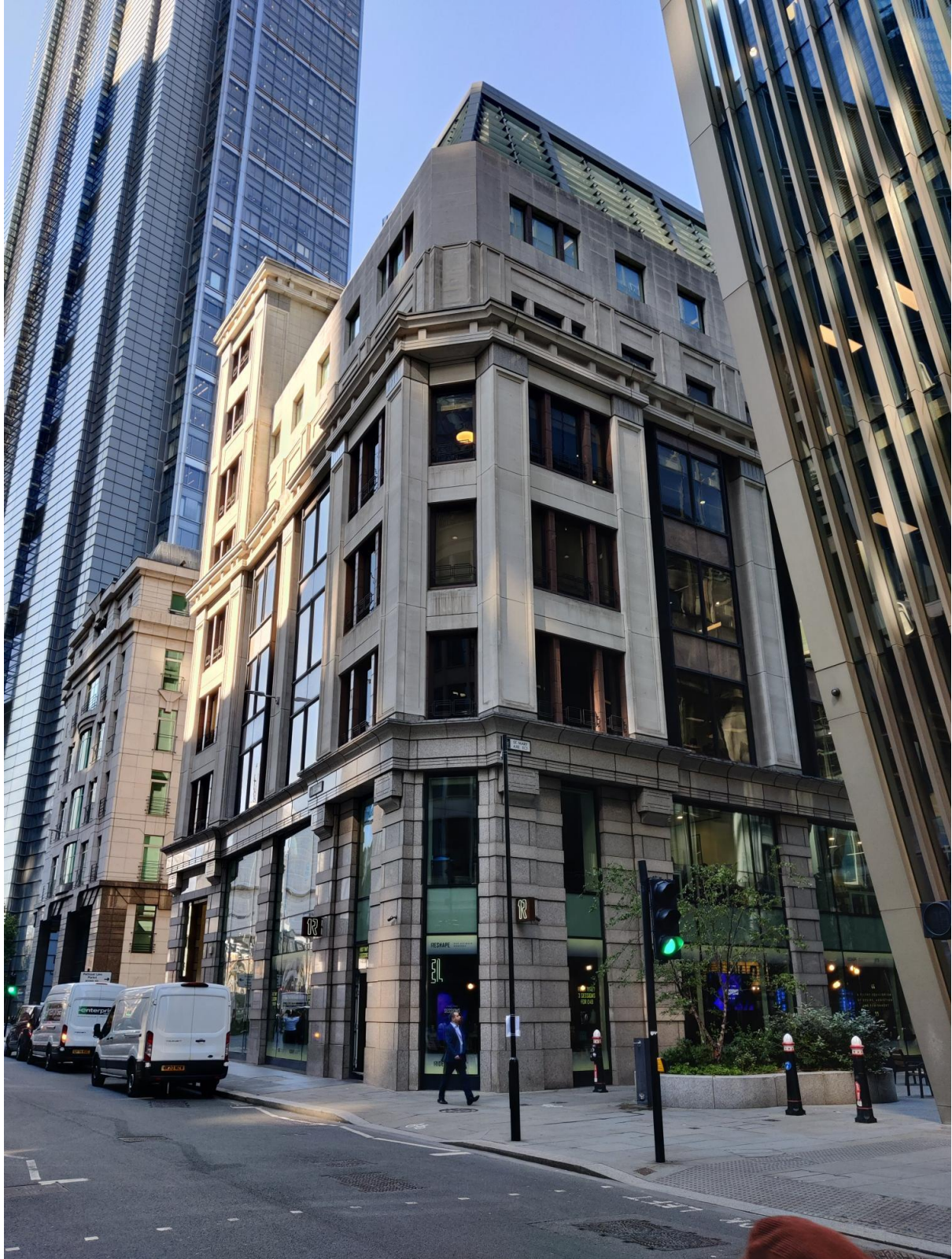
Existing view from southeast:
