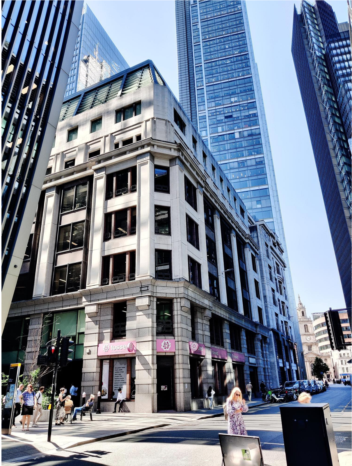
Existing view from north east:
