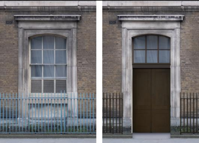
Image 1: Existing Window converted to a Door in West Wing to Provide Fire Egress
