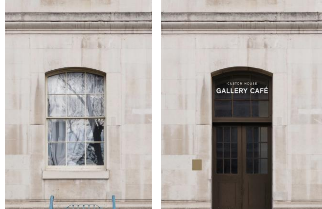
Image 2: Existing Windows converted to a Door in West Wing
