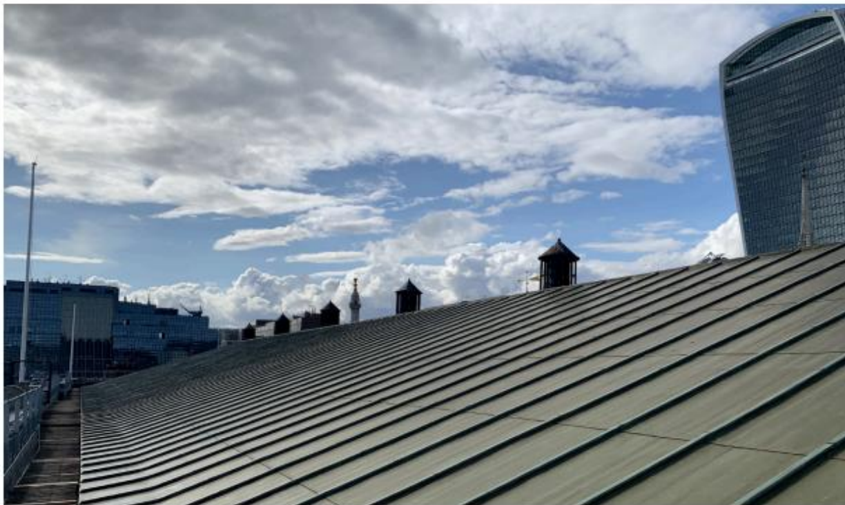
Image 1: Existing Central Copper Roof
