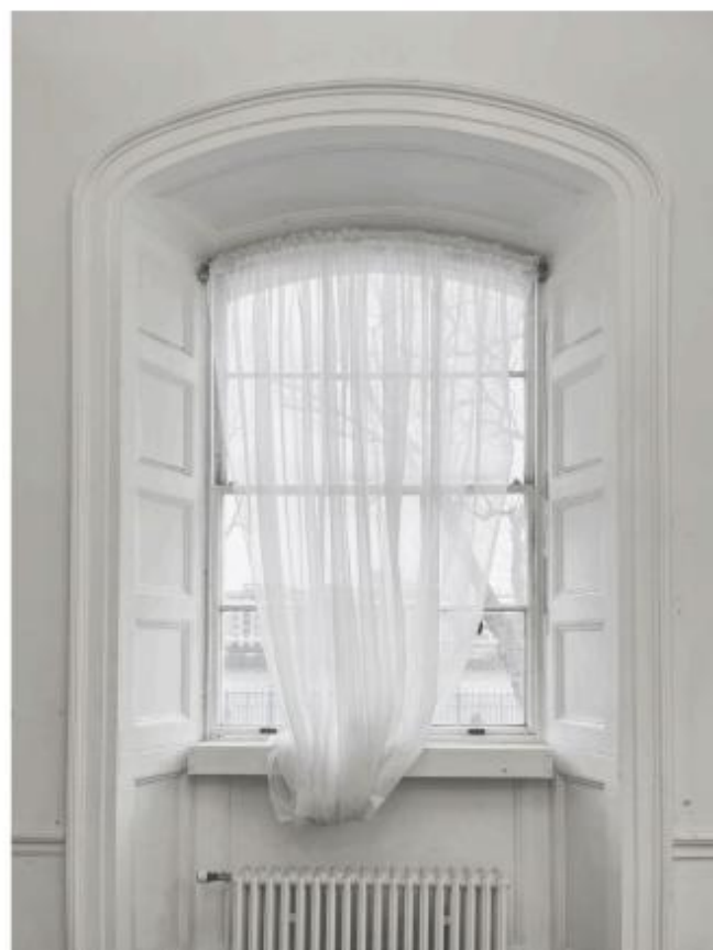
Image 1: Existing Window and Bomb Blast Curtains
