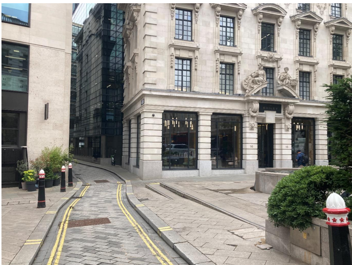
2025: 16 Old Bailey following completion of s278 works.
