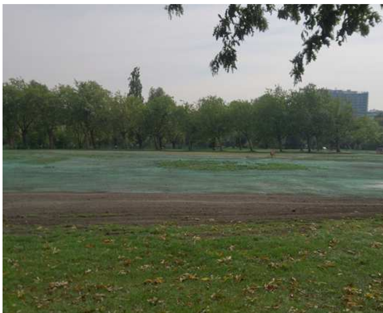
Hard standing following Hydro-seeding (September 2013)
