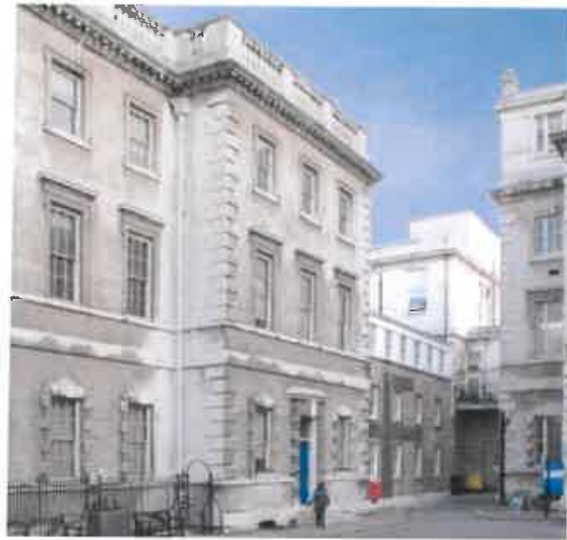
Finance Building, View from St Bartholomew's Square
