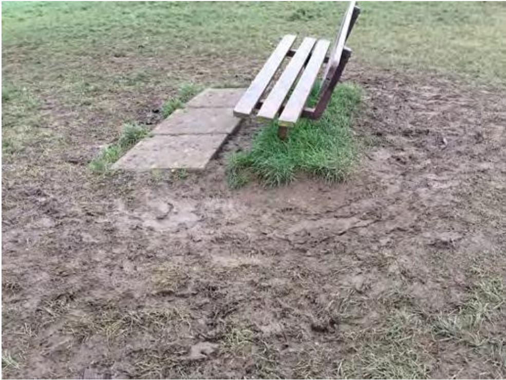
Figure 4: Grass Renovation Works, including deep compaction, levelling and post sward establishment
