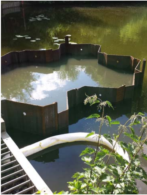
Picture 7—Temporary coffer dam at Viaduct Pond
