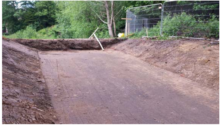
Picture 8—Spillway under construction at Viaduct Pond.
