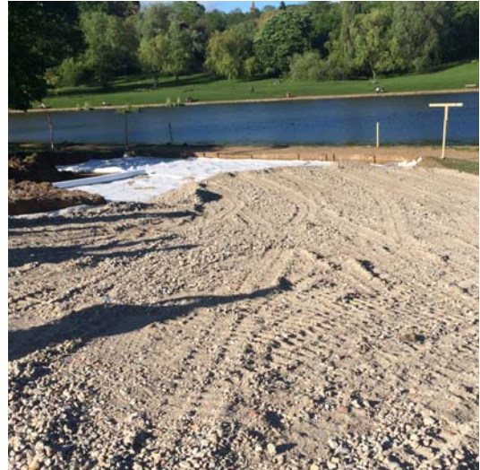
Picture 2 - Temporary crane platform under construction at Model Boating Pond.
