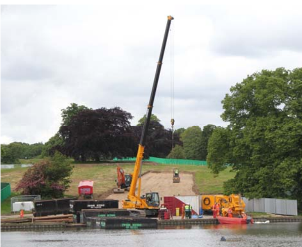
Picture 5 - Sheet metal piling at Model Boating Pond.
