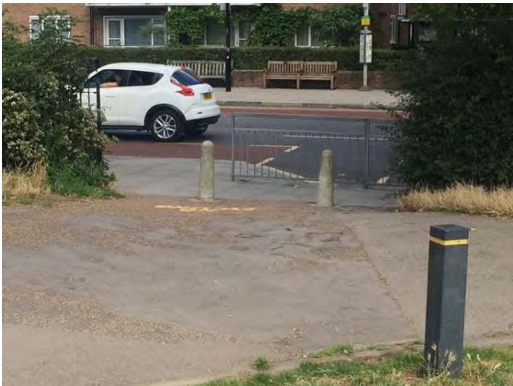
Figure 6 – Replacement of two concrete bollards with wooden bollards (Note 9, appendix 3 - proposed layout).
