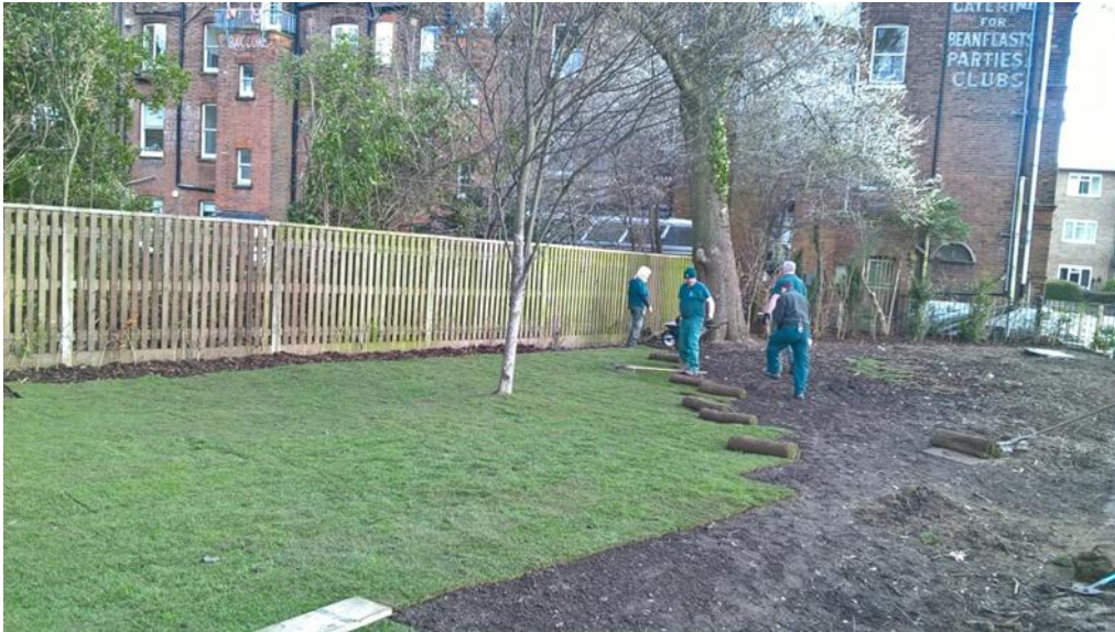
Figure 5: Swain's Lane landscaping works in progress
