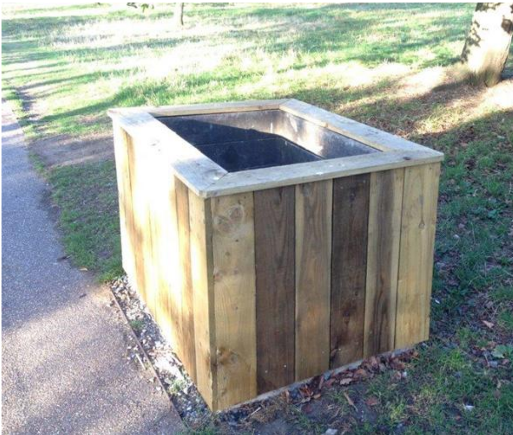
Figure 6: Bin with new wooden cladding
