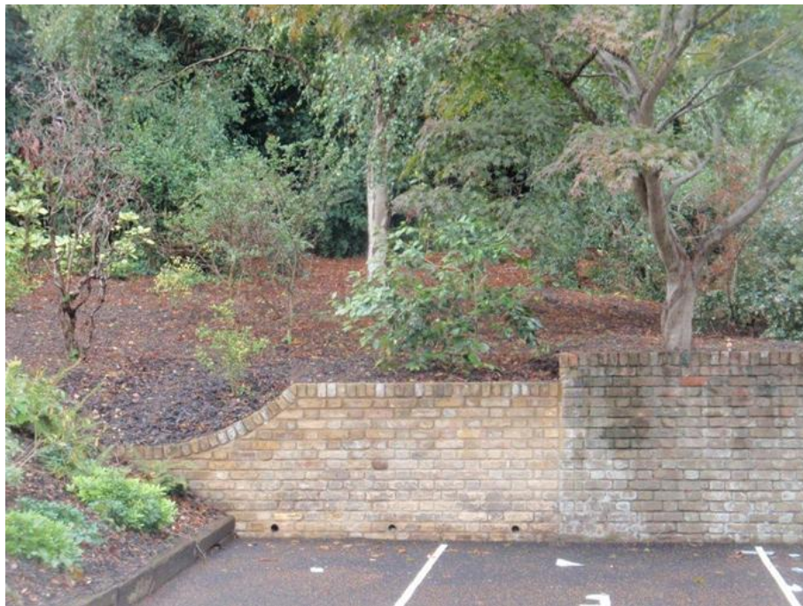
Figure 4: Disabled car park re-landscaping
