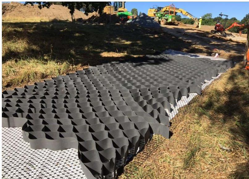
Figure 2: Anti compaction path section under construction
