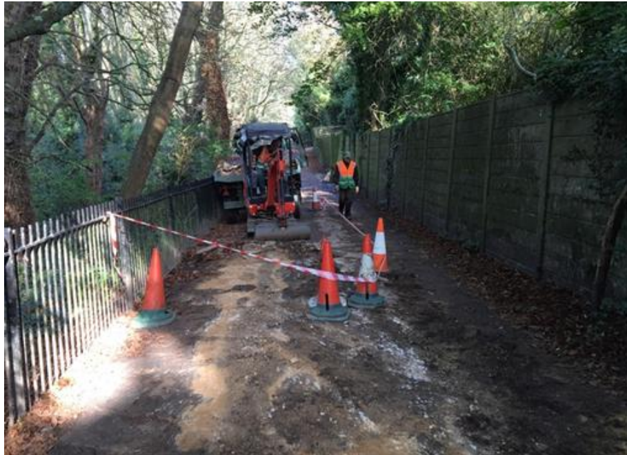
Figure 3: Conservation Team undertaking repairs to Millfield Lane
