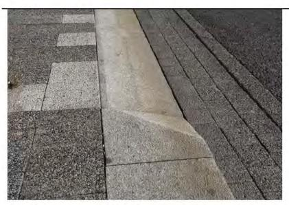
Dropping the kerb to a flush or very low upstand across the mouth of the motorcycle bays would reduce the physical separation between cyclists and general traffic lanes, potentially compromising the safety and effectiveness of the scheme. P2W users and other vehicles may be more likely to enter a cycle track with less physical separation when accessing the side roads or parking bays along Farringdon Street.
