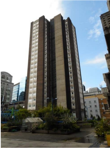
Middlesex Estate – 1 Tower Block
