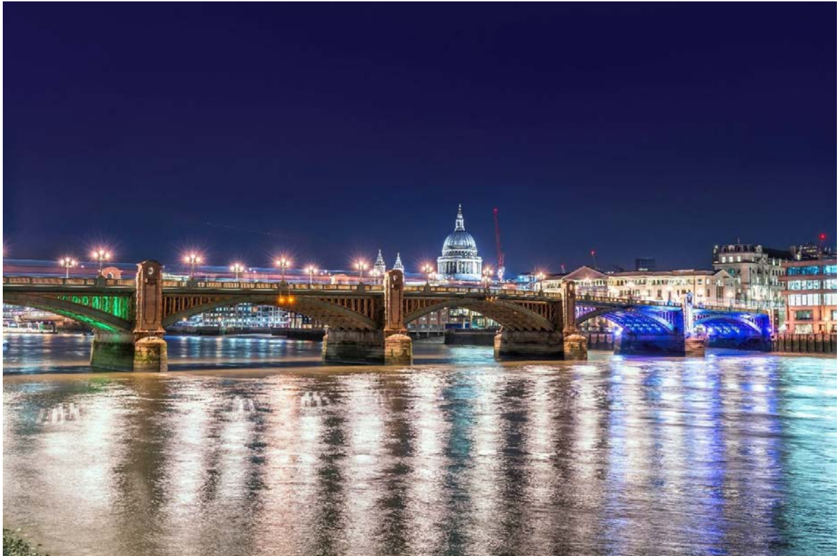
Southwark Bridge – Existing
