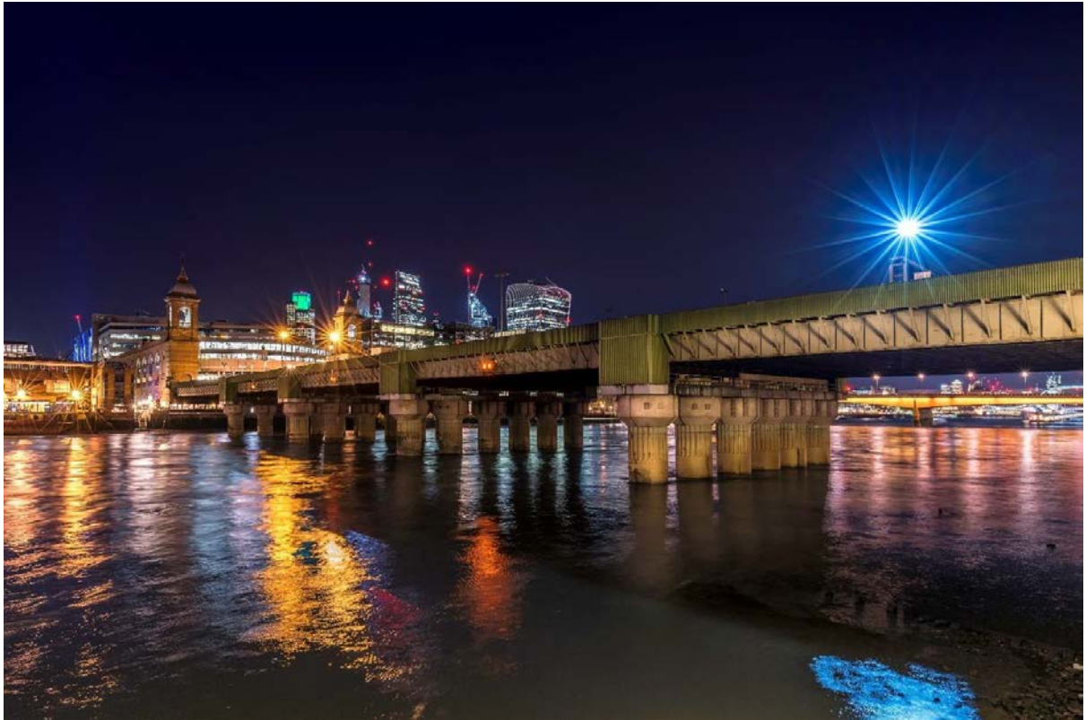
Cannon Street Rail Bridge – Existing
