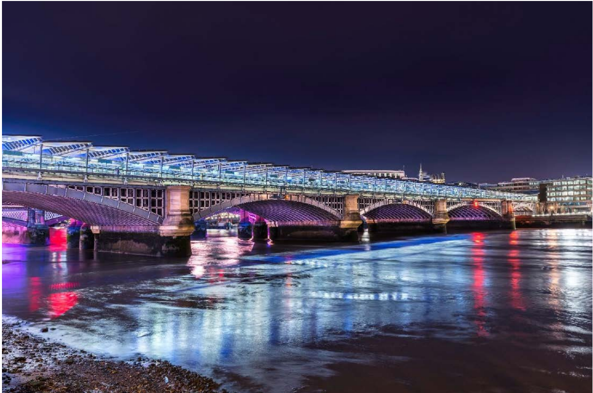
Blackfriars Rail Bridge – Existing
